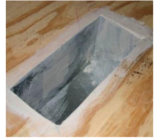
Sealed Register Boot
