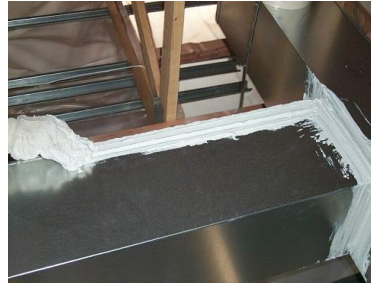
Sealed Branch and Trunk
