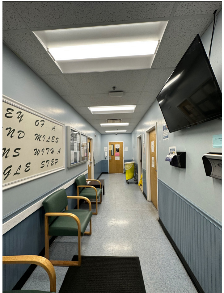
High Point Treatment Center upgraded 785 lighting fixtures and switches with LED lighting, sensors and dimmers. The project will help the nonprofit save 35% on energy costs—savings that the organization can put toward doing even more for the community.
